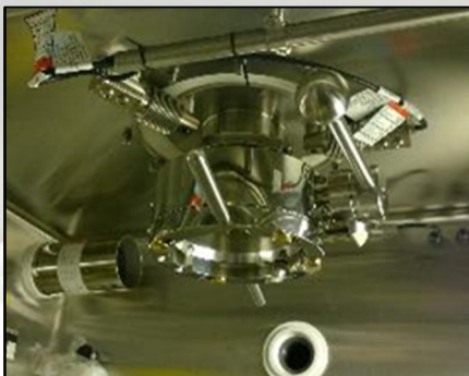
Weigh in Place
